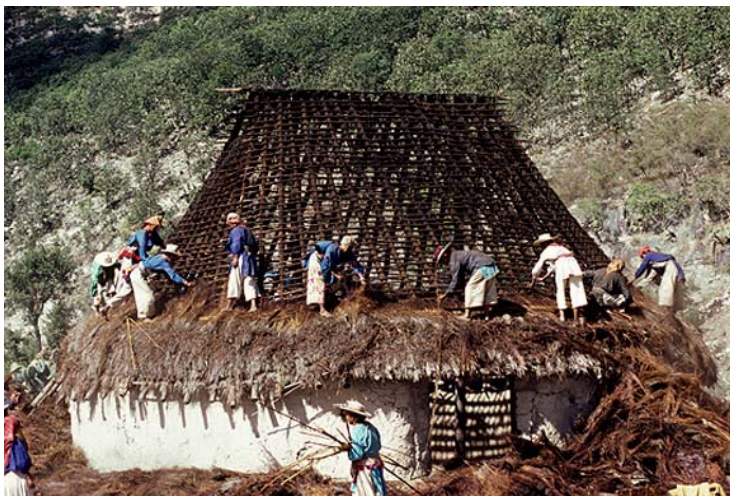
Renewing the Roof of the Tuki • Photograph © 1981 Juan Negrín
